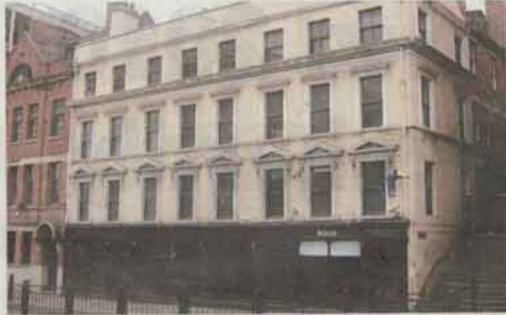
NEW THEME The former Julies Nightclub has plans in place.
